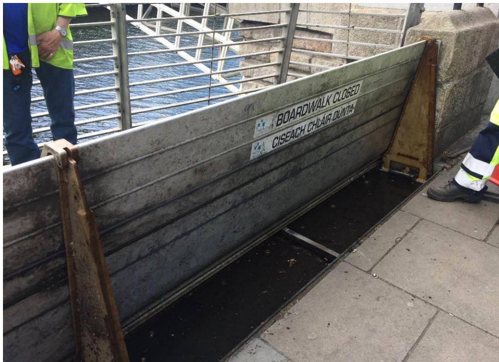
Fig. 29: Barrier in closed position
