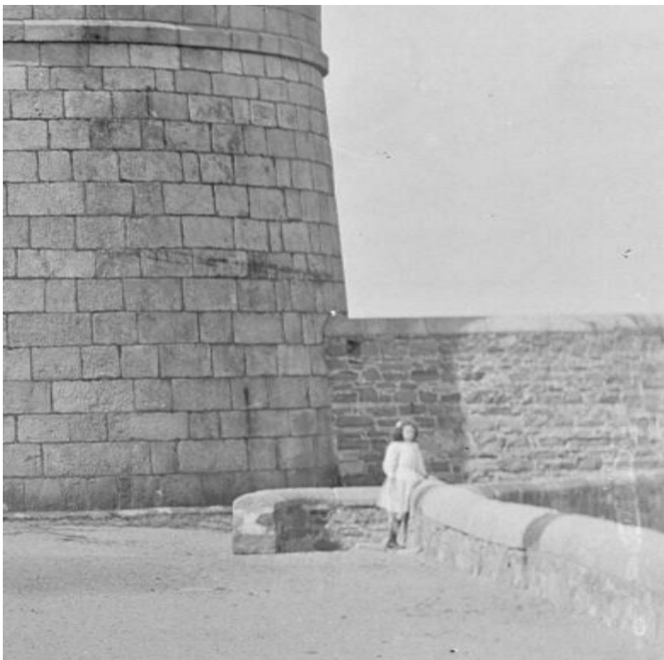
Fig. 15: Detail of previous image showing how the sea-wall joined the Martello Tower
